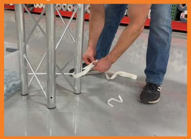
**9** Feed the anchor strap up to the ratchet and tighten it.
