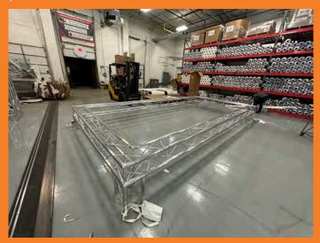
Lay out the canopy over the truss roof and lightly secure it to the corner using the ratchet straps so it doesn't slip off when adding the legs.
