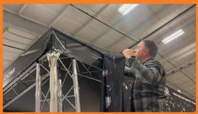
Wrap the edge of the wall around the truss leg using bungee balls. (Setup varies based on truss)
