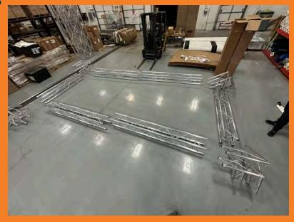
Assemble the top perimeter truss hardware first using quick clips or bolts to connect all the pieces.
