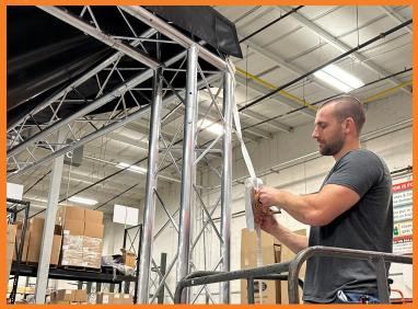
Connect the roof drain tubes directing them out the back legs and away from the tent.
