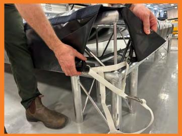
If you have a roof drain install the screw-in connectors on the underside of the roof, if they are not on the canopy already. Once installed leave this piece in place even when taking down the truss. Leg drain tubes should already be in the truss legs.
