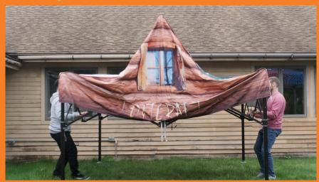
Stand by a corner of the frame, place a foot on the plate at the end of the tent leg (foot pad).
