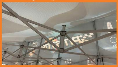
Holding the tent down with your foot on the foot pad, press up on the scissor piece attached to the corner bracket as it slides up the leg and clicks into place. Repeat for remaining legs.
