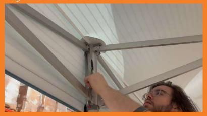
Pull on the strap to tighten until the valance itself is taut. Repeat for the remaining straps. (Remember to unbuckle these straps when taking the tent down.)
