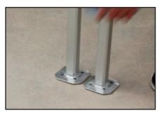
Set the two tents that are being connected next to each other so the baseplates at the bottom of the legs are almost touching.
