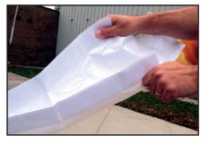
Unfold the rain gutter and locate the Velcro along both edges.
