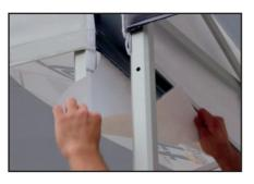
Fold the rain gutter towards the inside of the opposite tent and repeat the previous step to attach the second side of the rain gutter to the second tent.
